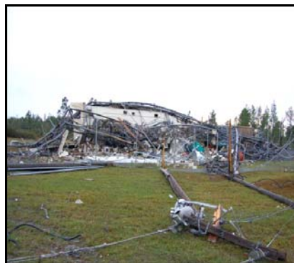
The Lake County Fire and Sheriff temporary transmitter site after the February 2 tornados.
